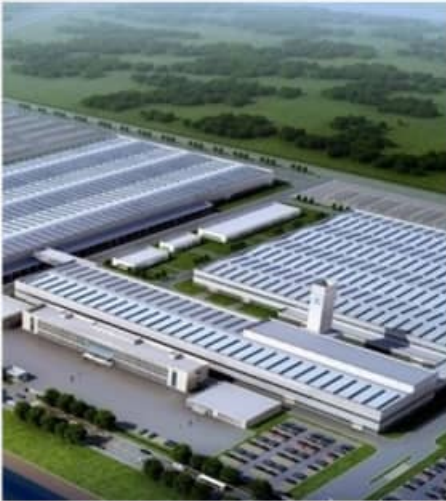
Adjacent to Tata Lithium Battery Plant
